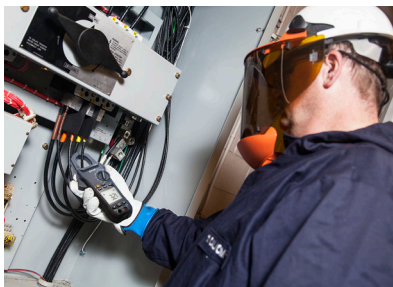
Analyze Power-related Issues
